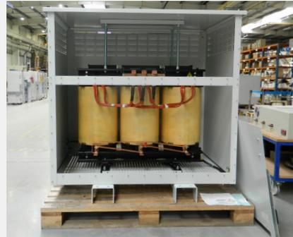
TRANSFORMER: ET3SM-630 440//690 dD0 60Hz T45F AL IP23
